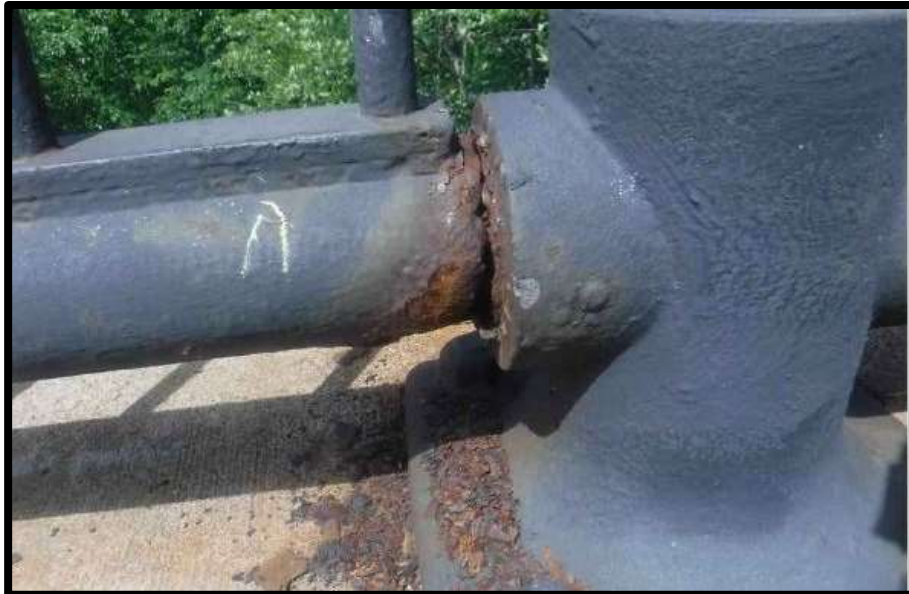
Deterioration at Pedestrian Rail
