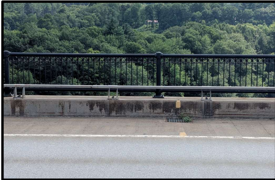
Existing Pedestrian Rail at Safety Walk
