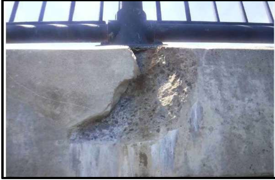
Spalling Concrete at Copings
