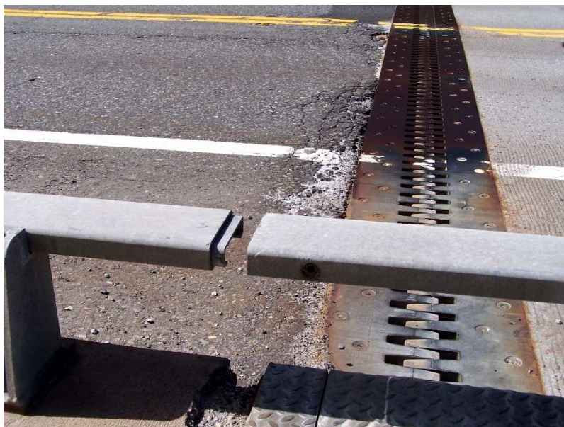
Potential Snag Point at Expansion Joint
