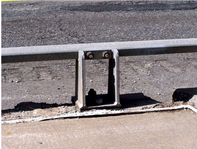
Spalling Concrete at Traffic Rail
