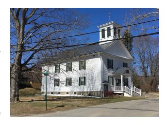
basement. The second floor consists of an open room used for town meetings and other gatherings. The building area is 3,901 square feet. The roof of the Town Hall was insulated in 2014 following a recommendation from the ASHRAE Level 2 energy audit completed by Bales Energy Study in 2014. This study also recommended replacing the heating system in the building. Additional insulation in the walls was completed in the fall of 2018 using funds from Green Communities competitive grant.
