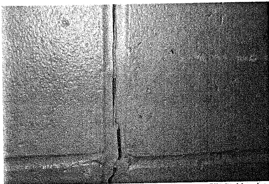
Gill Elementary: Cracks in expansion joint sealant are filled with paint.
