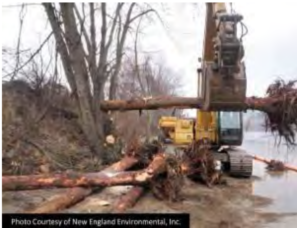
Photo Courtesy of New England Environmental, Inc. Construction of the large woody debris structure
