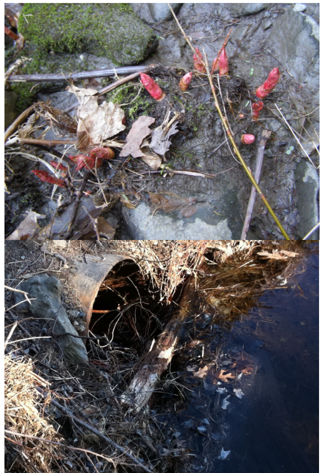
Top: Japanese knotweed emerging in spring. Bottom: Partially blocked culvert in area C.
