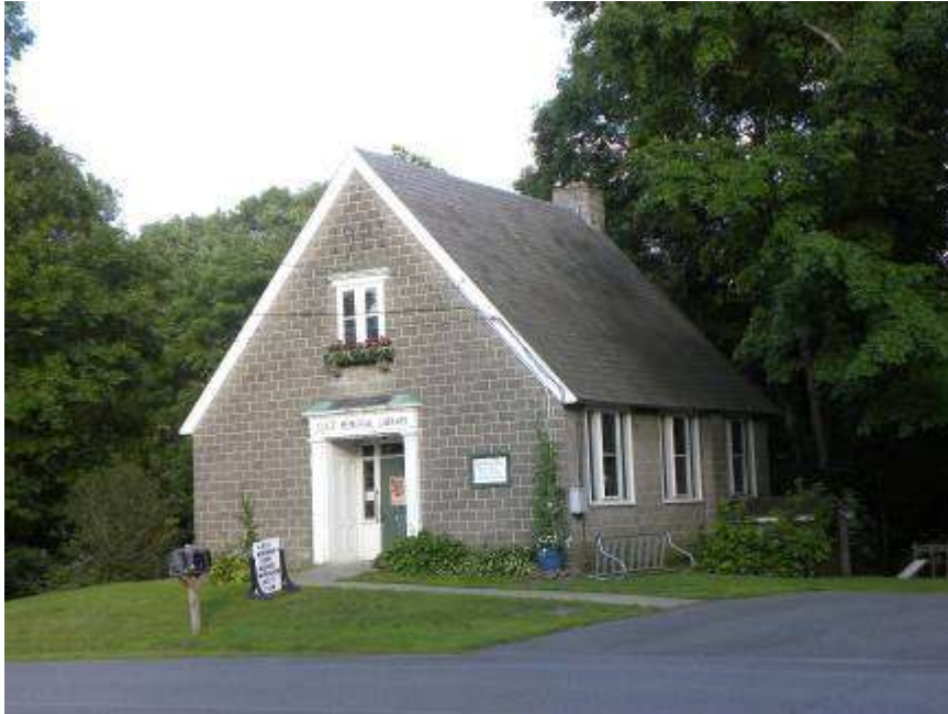
Slate Library is one of Gill’s twelve town-owned temporarily protected parcels.
